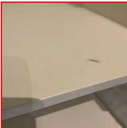
5.11.1 Marked and holes highlighted.
