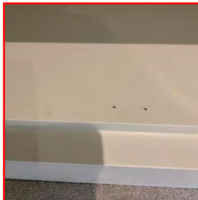
5.11.1 Marked and holes highlighted.
